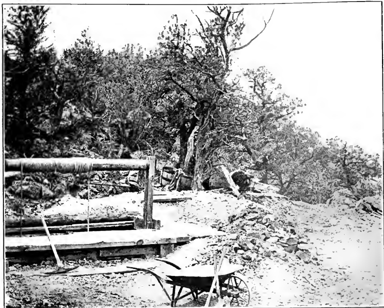
FIGURE 9. Shaft mining. Early method of raising quartz to the surface
