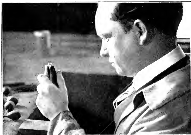
FIGURE 93. Seeing that the stone is level
